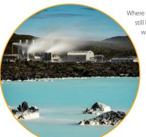
Where heated water does not naturally reach the surface of the earth, it may still be close enough to the surface to allow access through drilling. Even where there is no hot underground water, geothermal energy can be created by drilling a hole for input of water into the heated rock, which is then turned into steam and released through a second output hole to allow for electricity generation.
